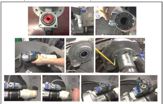
7. Connect gas and electrical supply to water heater and check for gas leaks. Adjust the CO<sub>2</sub> percentage to the appropriate model data given in Table 1 when water temperature is 55°C. Turn the venturi screw clockwise to increase CO<sub>2</sub> percentage, and counterclockwise to decrease CO<sub>2</sub> percentage.
