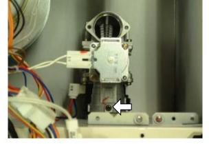
(2) Pull up the gas electromagnetic valve to the upper section and remove it.
