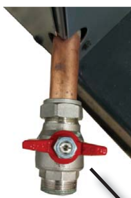
Tank drain shutoff valve
